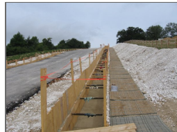
Bramley - Didcot 400kV Cable Replacement Scheme
