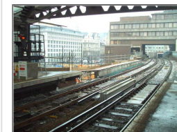
Blackfriars Thameslink Project - Temporary Rail Bridge
