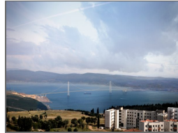
Izmit Bay Crossing
