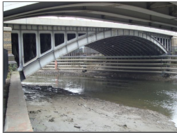
A13 River Lea Bridge Replacement
