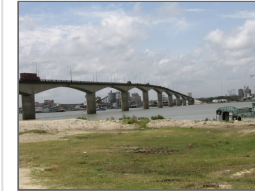
Seismic Assessment and Retrofit of Meghna & Gumti Bridges
